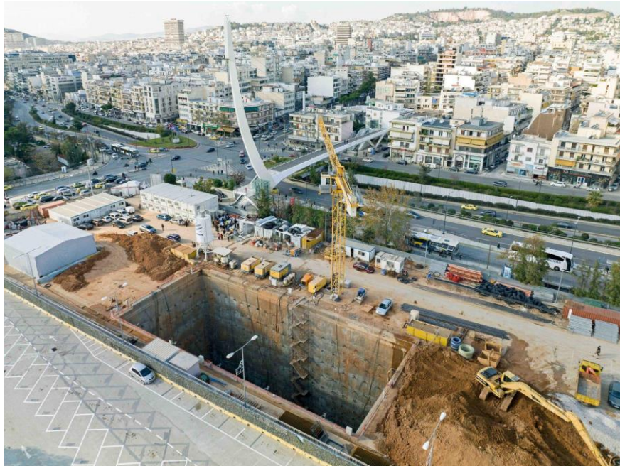
Athens Metro Line 4, under construction: Katehaki TBM Shaft (photo: www.ametro.gr )
